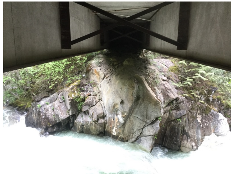
Left Bank Abutment when facing downstream
