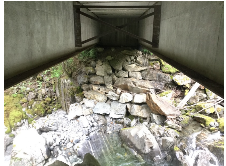
Right Bank Abutment when facing downstream
