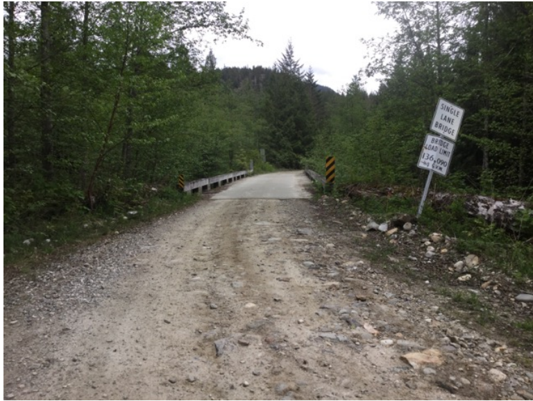
Approach from Right Bank when facing downstream
