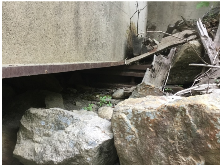
Downstream left bank footing
