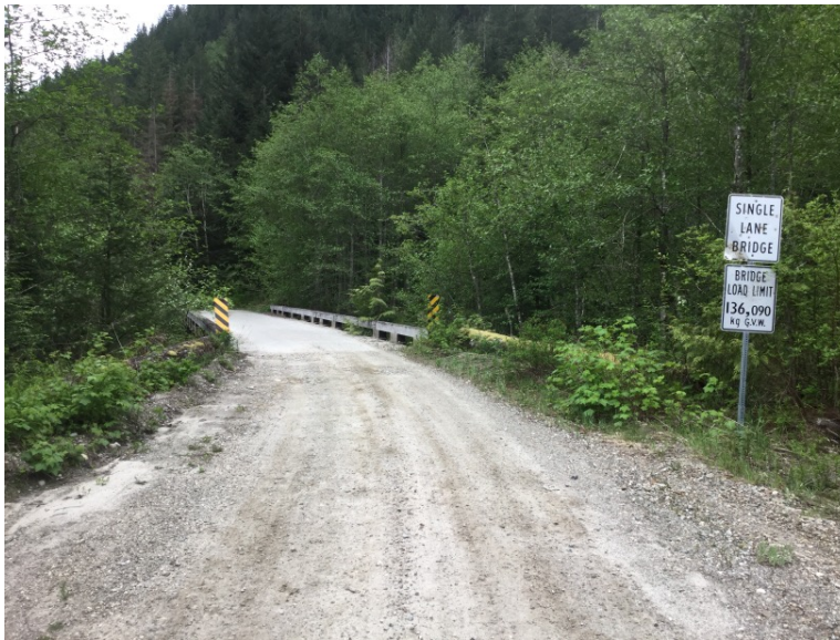
Left Bank Abutment when facing downstream
